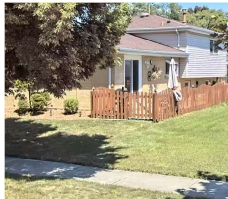
Fence encroaching into front yard
